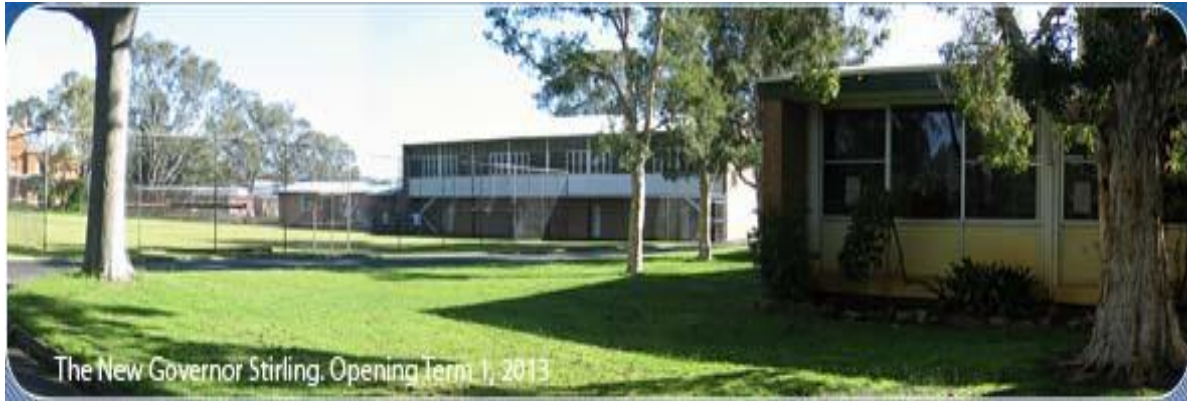
The Squash Courts and the western end of the Library
